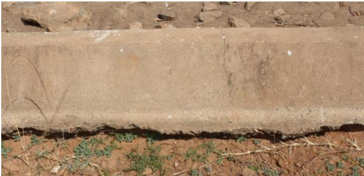
Figure 24: Undercutting of service spillway outfall sections across full length.
