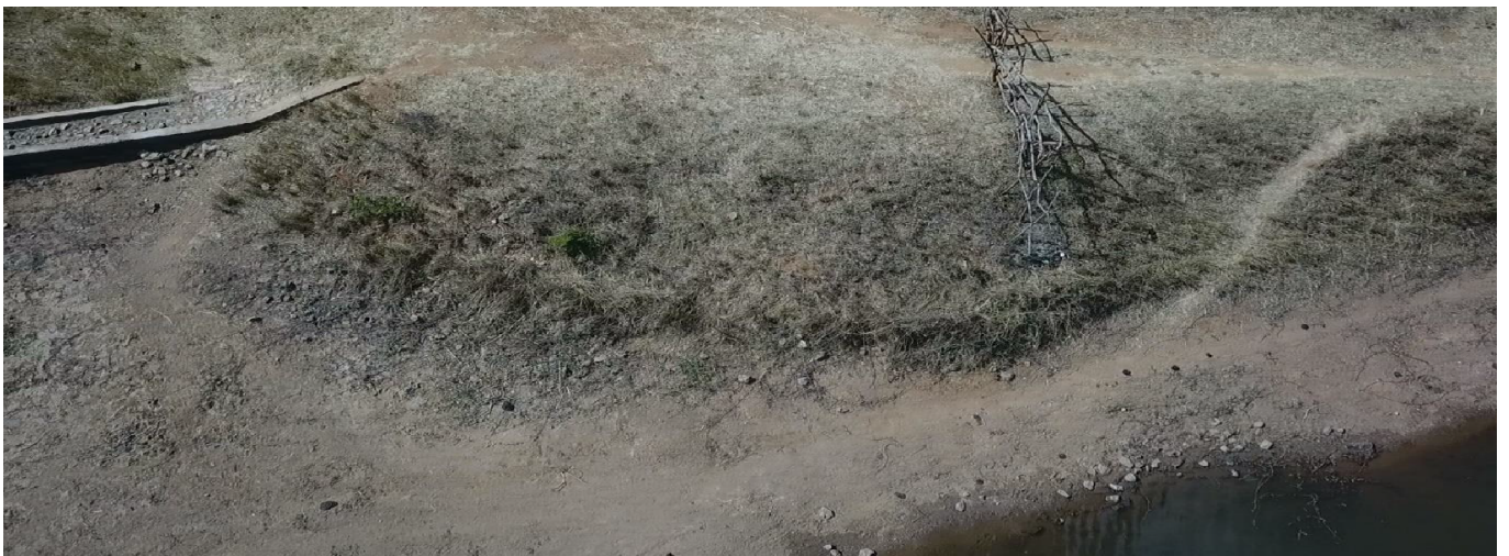
Embankment bend at spillway – paths and minimal stone pitching.
