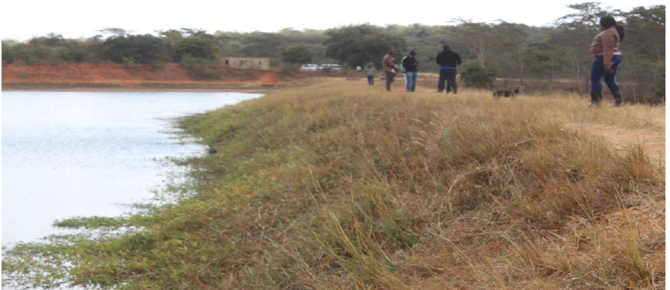
Front face from right bank showing variation in embankment slope
