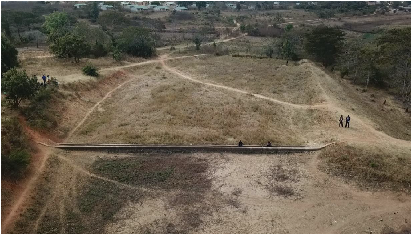
Service spillway and return channel
