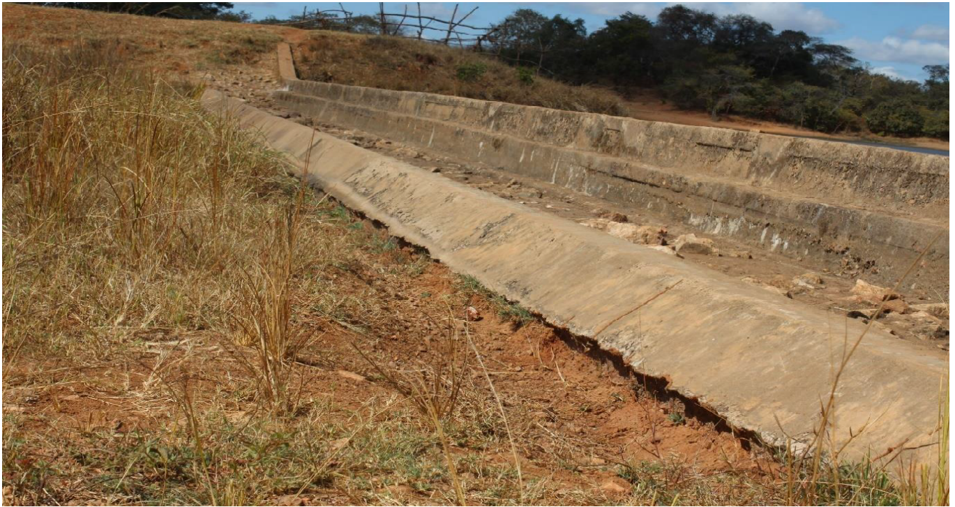
Service spillway showing signs of undercutting
