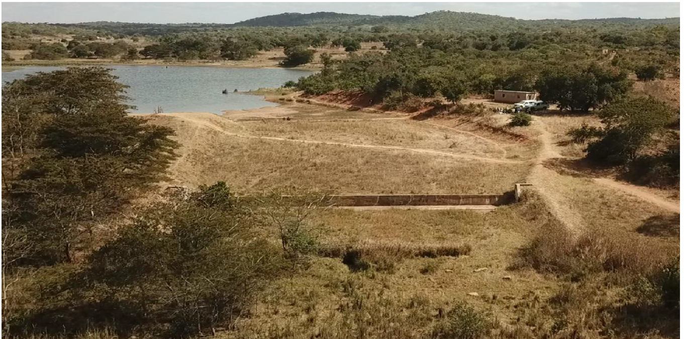
Spillway return channel and drop structure from outfall end
