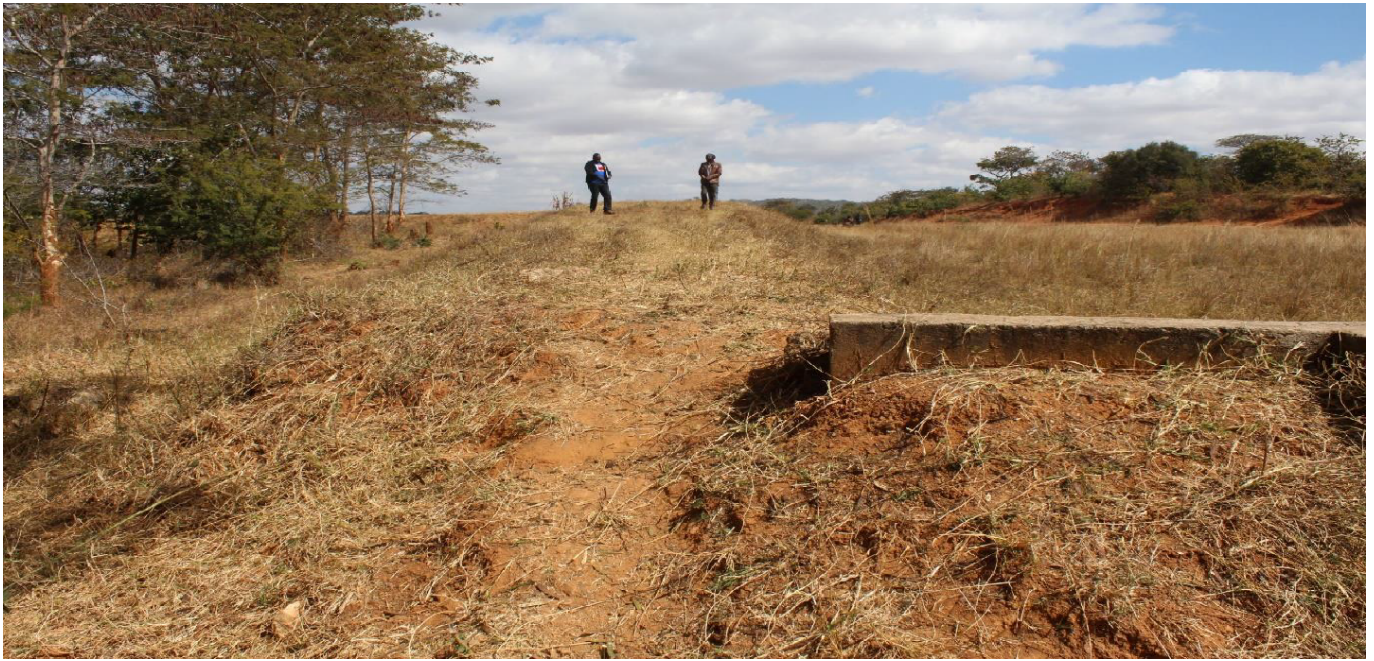
Right bank training wall and drop structure abutment
