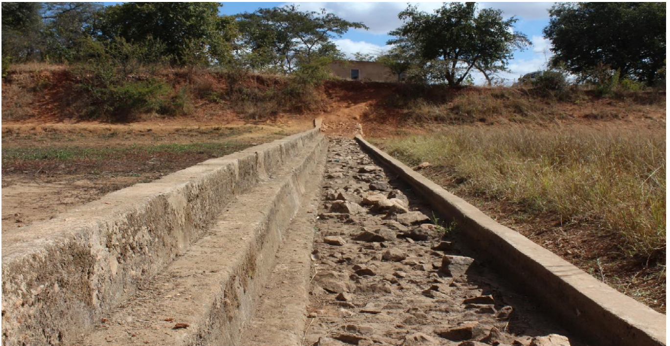
Service spillway showing sill, dissipator and minimal left-hand abutment
