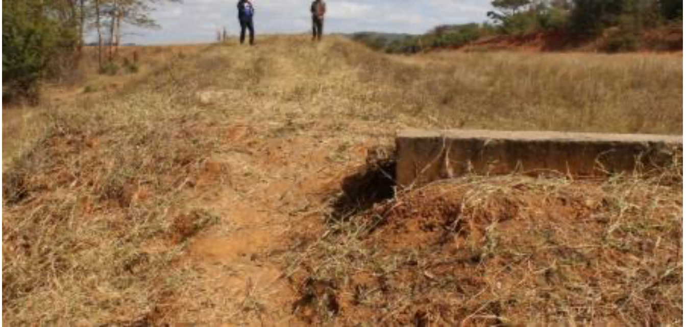
Figure 27: Right hand drop structure abutment showing potential for bypassing
