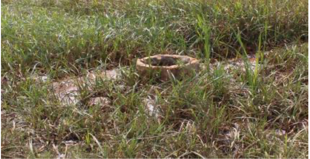
Figure 28: Circular masonry valve chamber in seepage area
