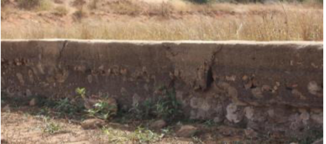
Figure 21: Condition of upstream face of service spillway sill section
